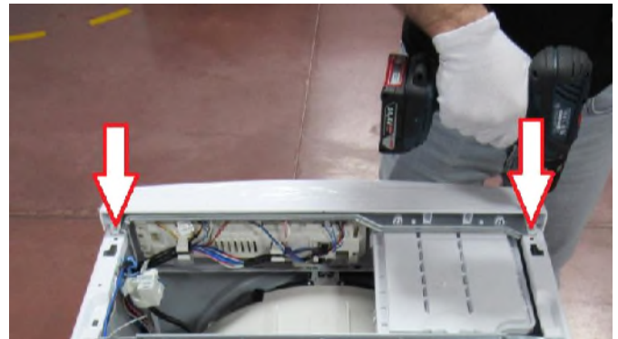
4.12 Tighten two screws fixing control panel.
