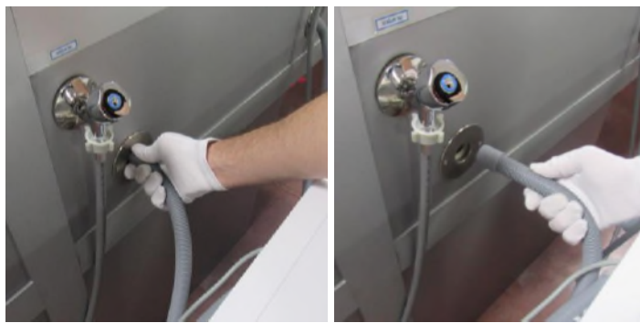
1.3 Disconnect the drain hose
