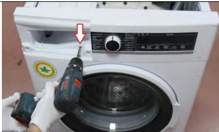
3.11. Tighten the screw which fixes the control panel to the front panel.
