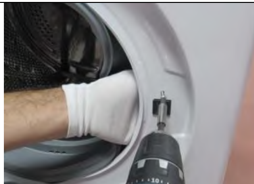
3.6. Tighten the door lock screw
