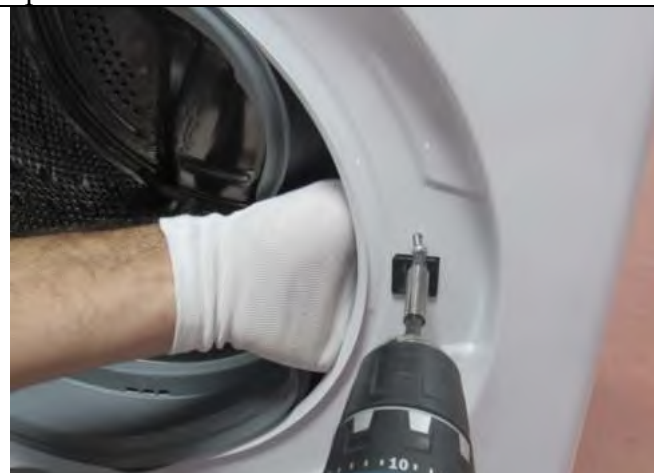
3.5.1 Tighten the door lock screw
