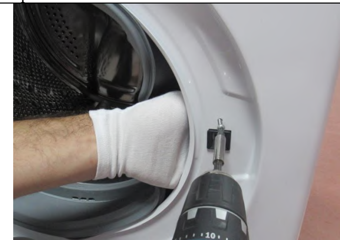
3.5.1 Tighten the door lock screw
