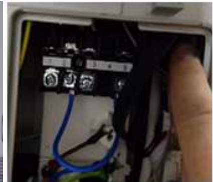
Energize the air conditioner by pressing the on/off button on the indoor unit board.
